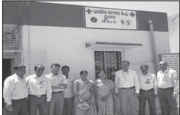
Primary Health Centre at Luwara village, Dahej
