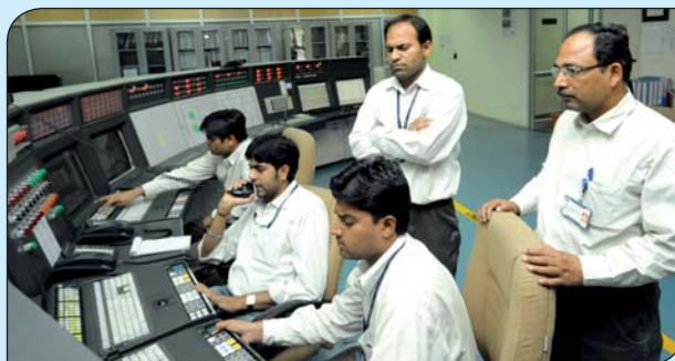
Employees at Control Room - Dahej LNG Terminal
