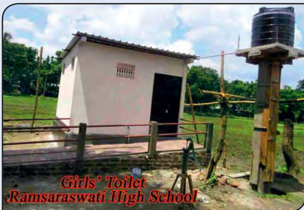
Construction of Girl's Toilet in Assam.
