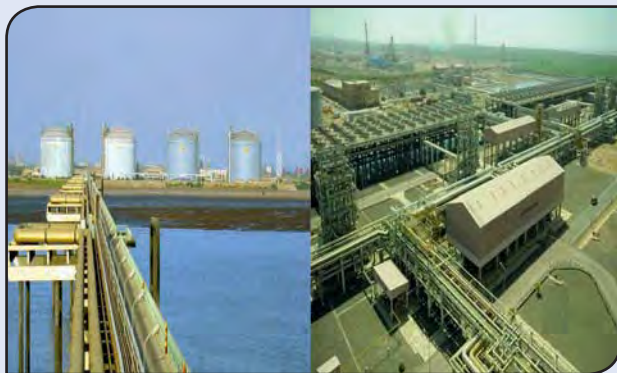
Expansion at Dahej Terminal
