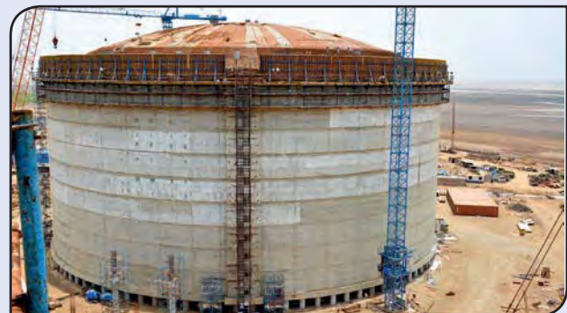
Expansion at Dahej Terminal
