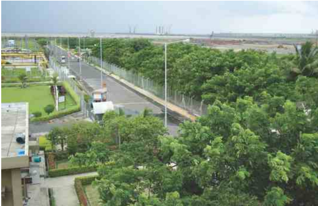
Plantation in & around Dahej Terminal
