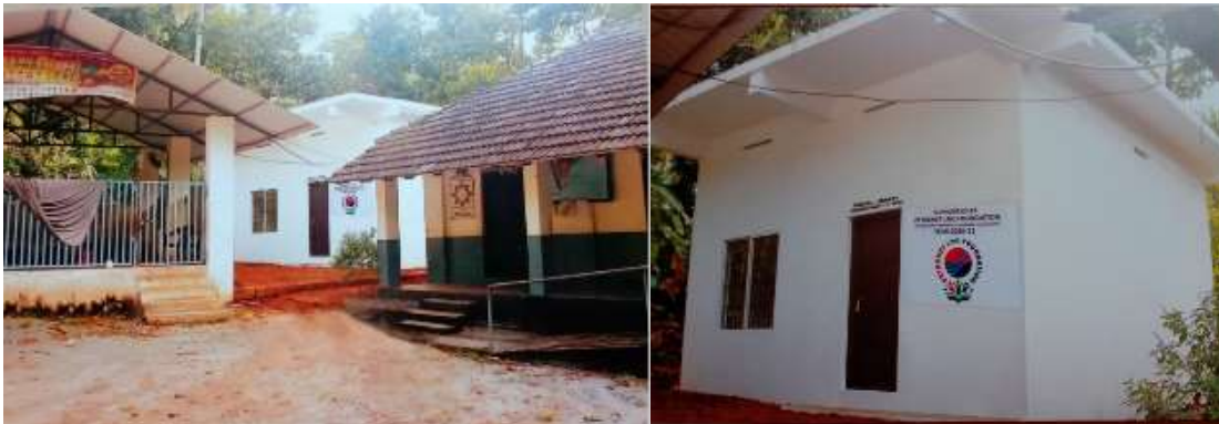
Construction of School library for Arumughavilasam LP school, Kannur
