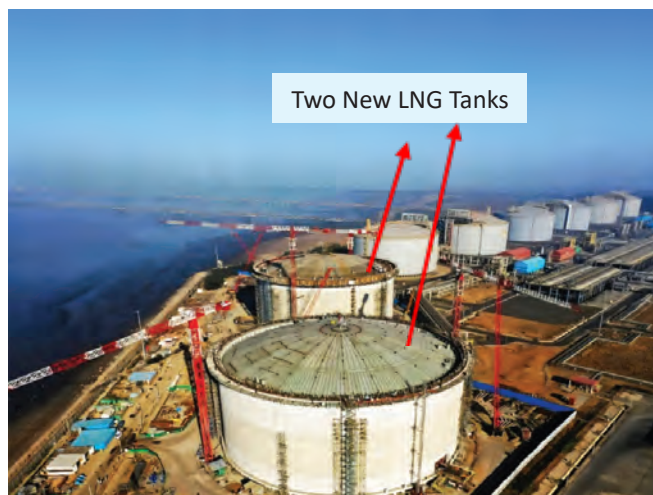
Two numbers New LNG Storage Tanks under construction at Dahej
