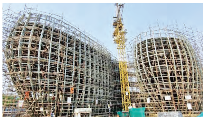
Construction of office complex at Dwarka, New Delhi
