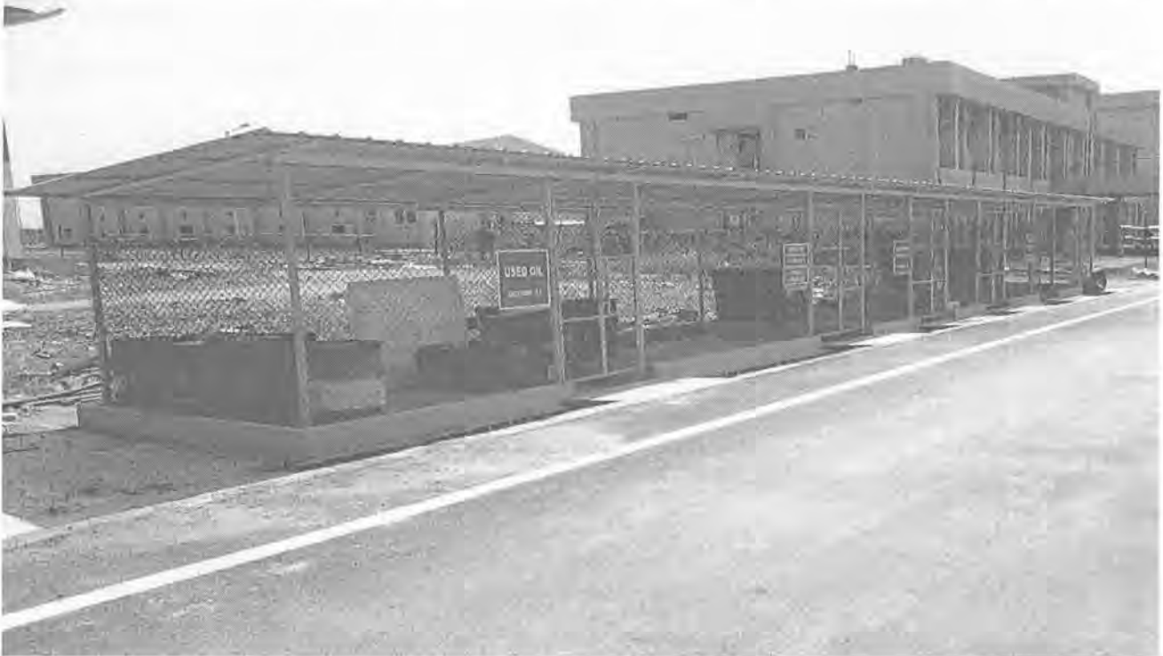
Fig-1: Hazardous waste storage facility.
