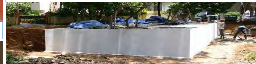
Completed Water Tank at Fort Kochi Parade Ground
