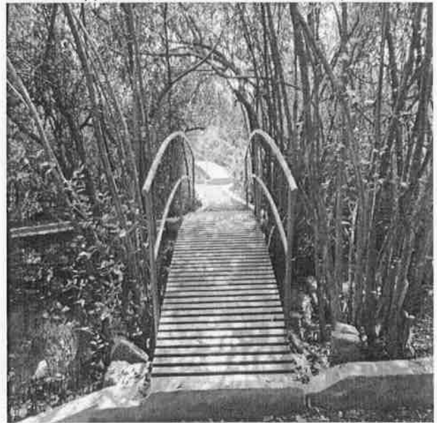
Inside view of Park (II nd and III rd bridges)
