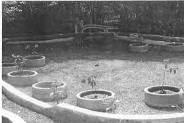
A view of mangrove demonstration garden at Malippuram (work in progress)
